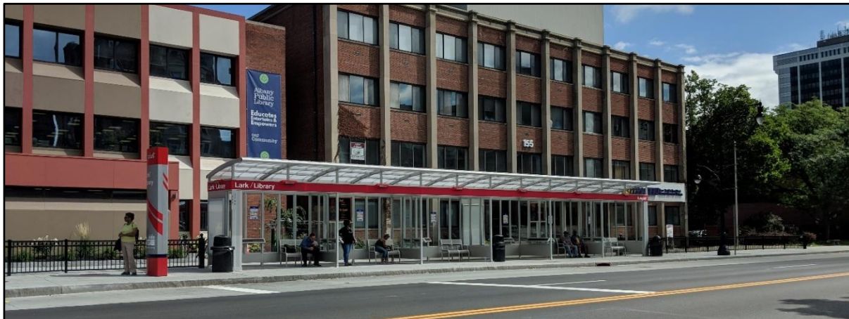
Completed Westbound Lark/Library Station shelter and pedestrian infrastructure.
