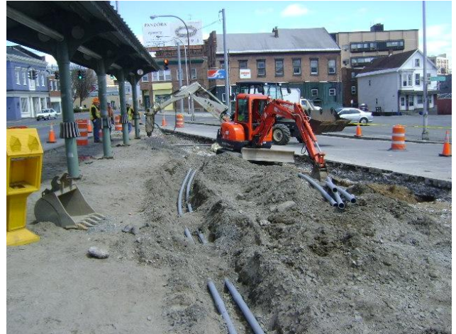
Liberty Park excavation
