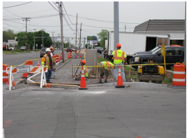
Setting the curb at Woodlawn Plaza
