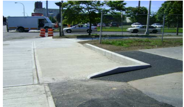
North Manning eastbound on Central Avenue
