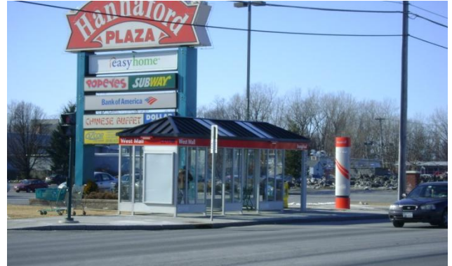
The prototype installation
