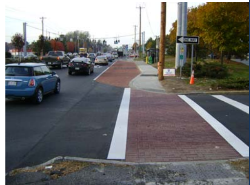
New high visibility crosswalks
