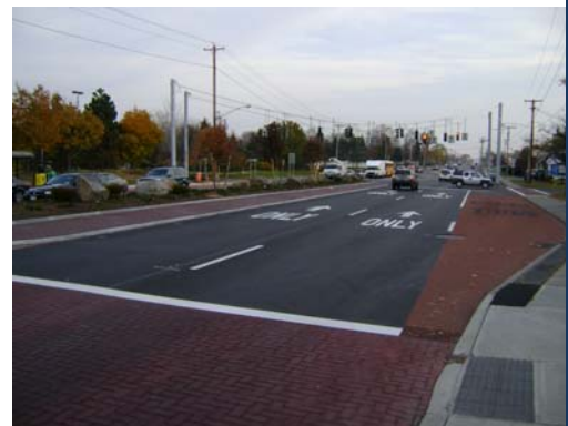
The raised landscaped median in Colonie was made possible through cooperation and partnership of the Town of Colonie, NYSDOT, and CDTA. Thank you!
