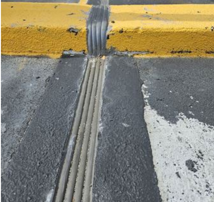
JLB Top Deck Joint Replacement
