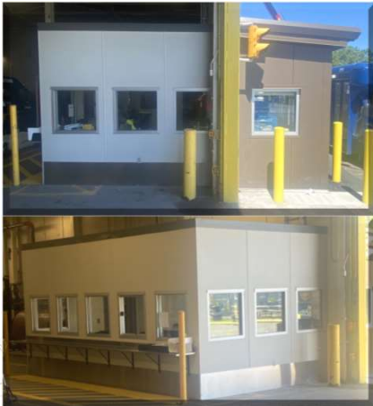
Replace Foremans Office
